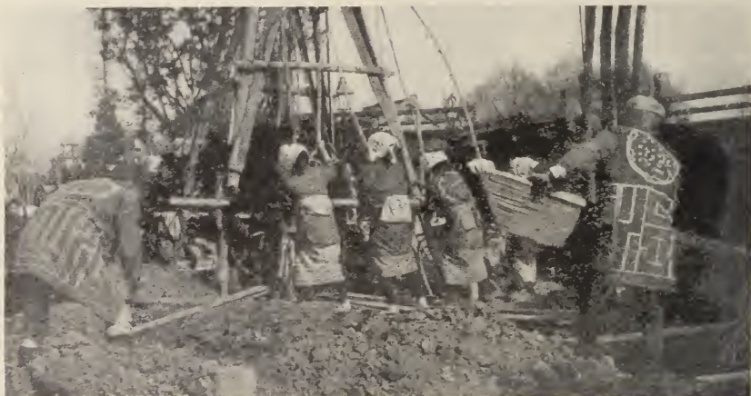
WOMEN DRIVING PILES FOR A FOUNDATION
